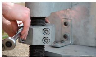
Use 3/8 hex to tighten socket screws in a cross pattern until the specified torque is reached.
