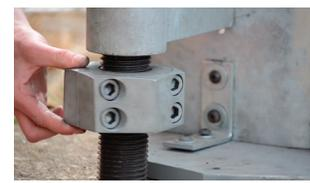
Twist the split nut up to the base plate component and tighten down the structural nut at the top of the base plate component
