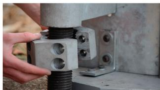
Place both halves of the nut around the anchor rod and align edges.
